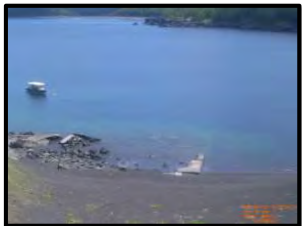
Photo 3.13-4. Current Condition of the Pagan Pier
