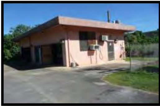
Photo 3.14-3. Maui Well #2 Pump
