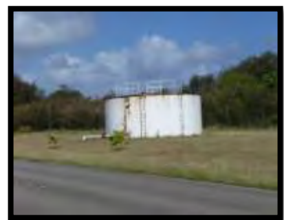
Photo 3.14-7. Tinian Airport Potable Water Storage Tank (60,000 Gallon Tank)
